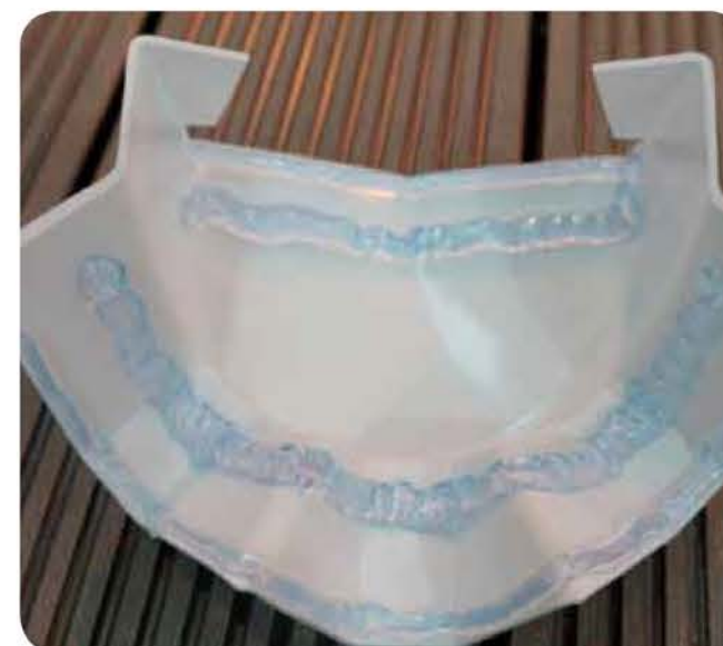
19 Using a suitable high grab adhesive sealant, run a small bead on the perimeter edges and a larger bead further inboard as shown. Recommended sealant is Soudal Fix All Super Clear.
