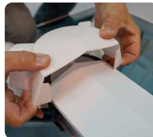
20 Splay the top cap and lower onto the ridge whilst checking the capping is positioned correctly over the rafter and hip top caps. The capping returns should clip under the ridge profile when positioned correctly.
