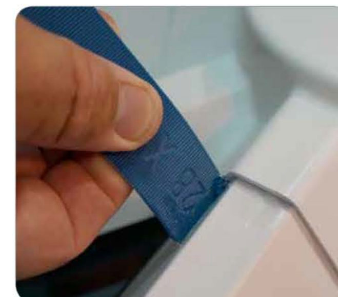
21 Ensure the capping is seated down correctly and remove any excess sealant from all edges.
